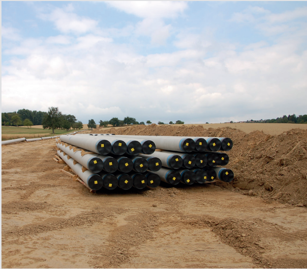
Figure 2: Pipes for the field test section, with barcode labels at their ends
